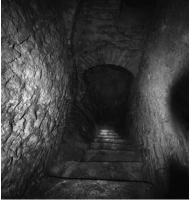
5 Ravne njive tunnel stairway. – After MARASOVIĆ/PEROJEVIĆ/MARGETA 2014 (note 7) 170 fig. 10.
