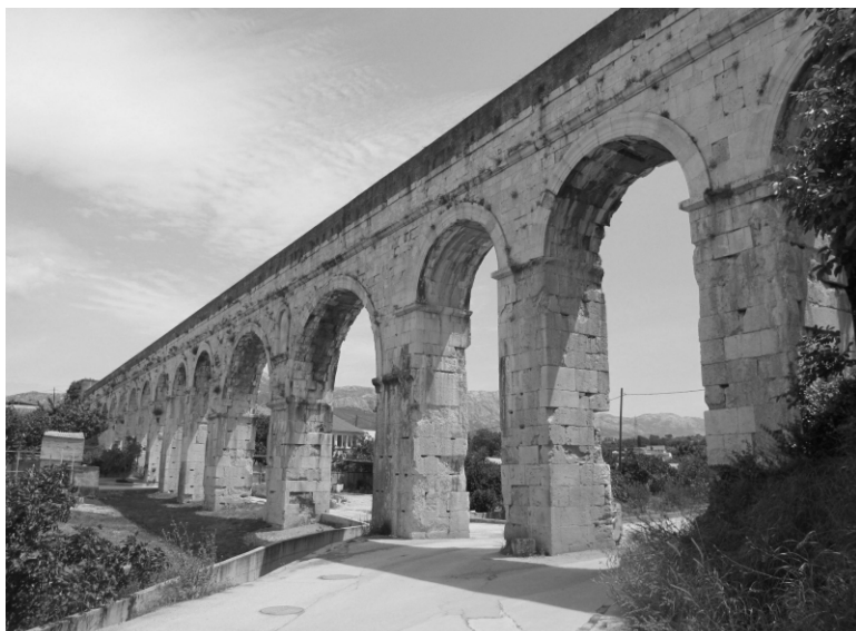
3 Columns and arches of the aqueduct at the site called „Dry Bridge“ in Mostine. – http://www.romanaqueducts.info/aquasite/split/foto14.html .
